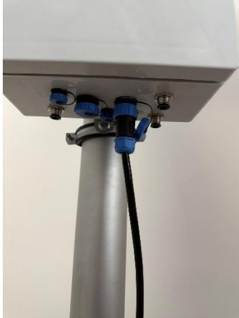
Connection to the mast
